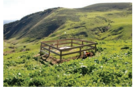
Utility enclosures to exclude cattle should be of a common design
