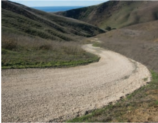
Shale and similar permeable base roads are compatible with wildlife corridors and cattle operations.
