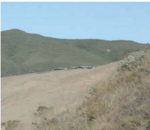
Low roof forms and low profile building mass
